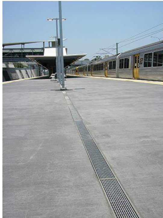
Figure 75: Linear Trench Drainage
