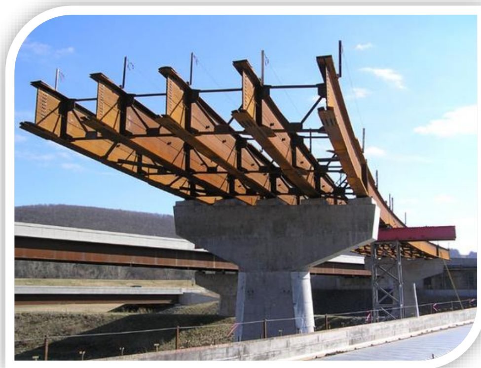
Figure 10 - Steel Girders (Source: Haskins, M 2015)
