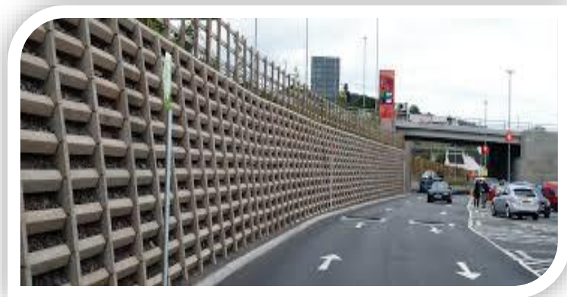
Figure 39 - Concrete Crib Wall
