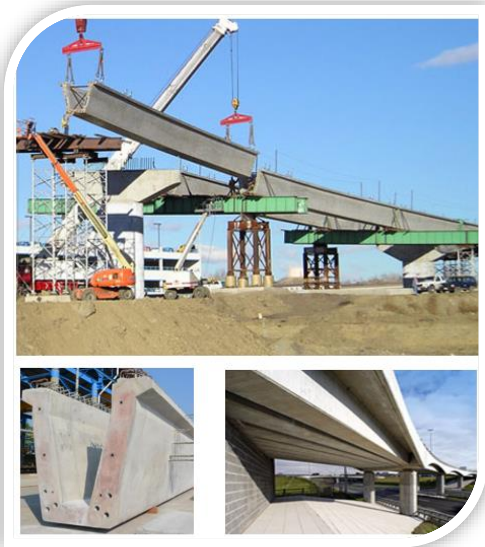
Figure 8 - Precast Super Tee Girders (Source: Sumit Engineering Group, 2010)
