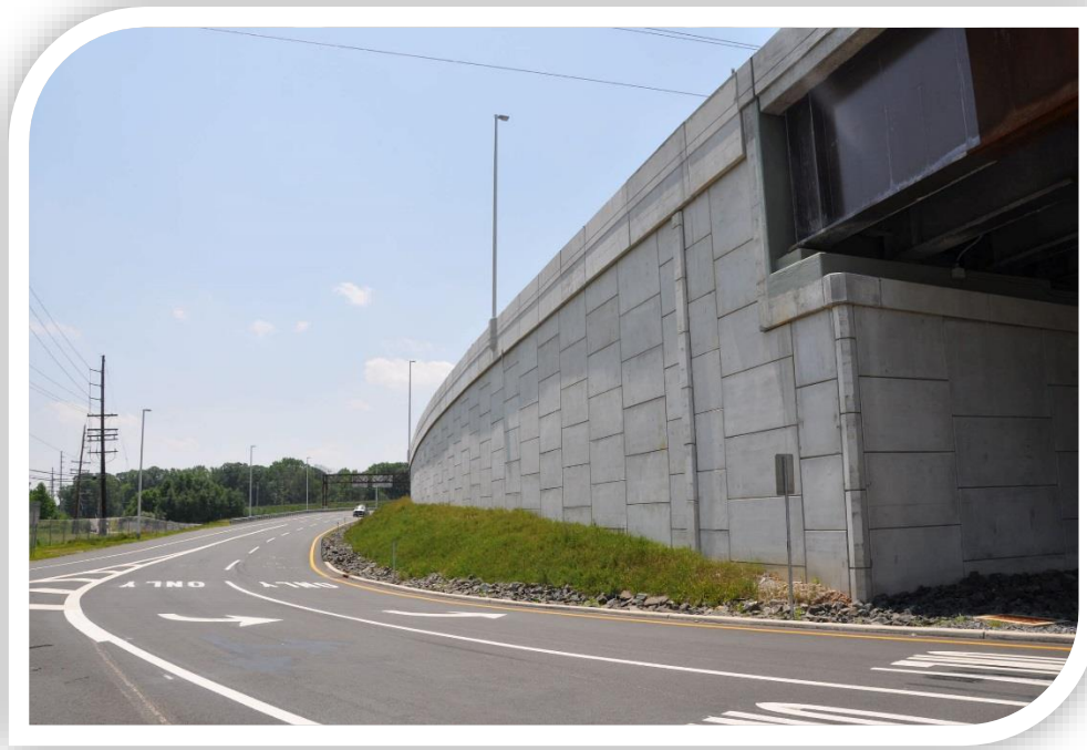
Figure 40 - Mechanically stabilised Earth Wall (MSE)
