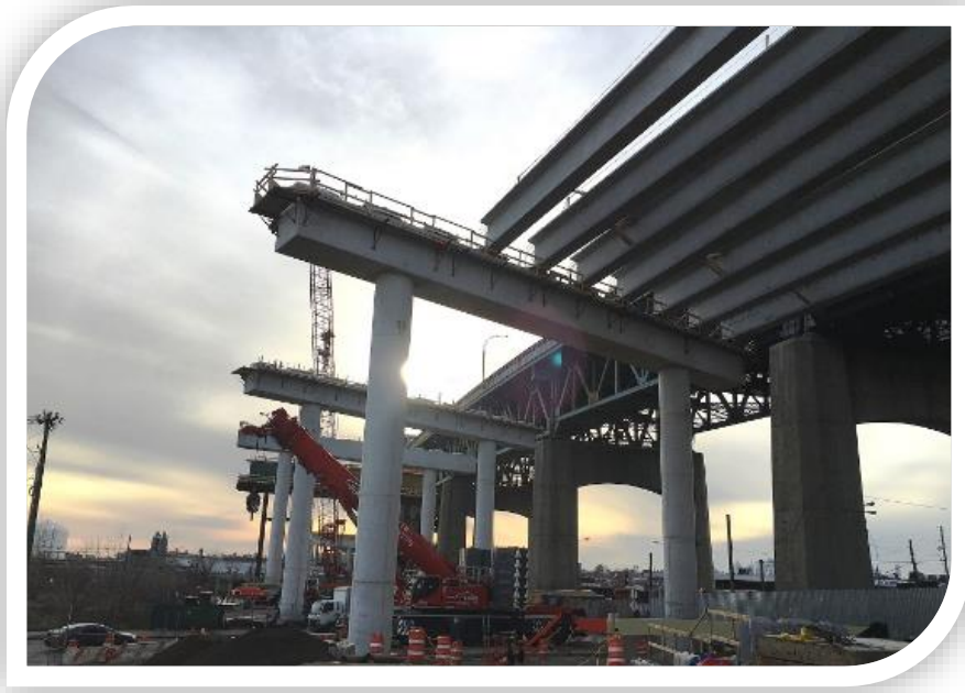
Figure 28 – Girder structural System
