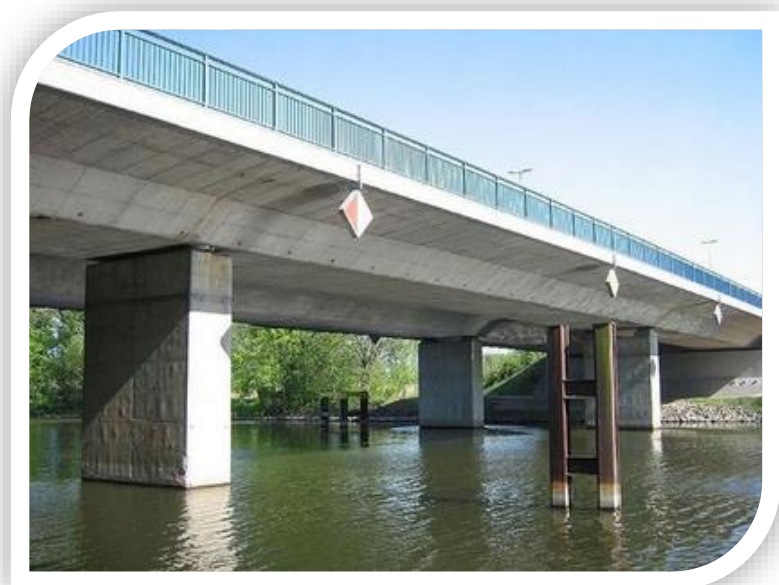
Figure 9 - Precast Reinforced Girders
