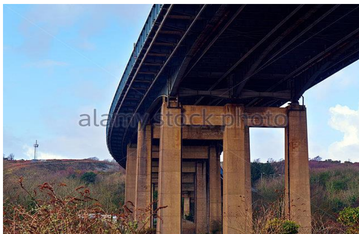
Figure 13: An example of square reinforced concrete columns
