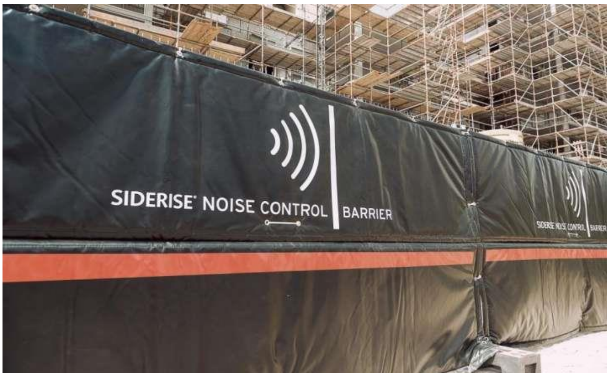
Figure 12- Noise Barrier (Heras 2017)
